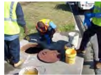
Figure 2: Removing a catch basin manhole lid
